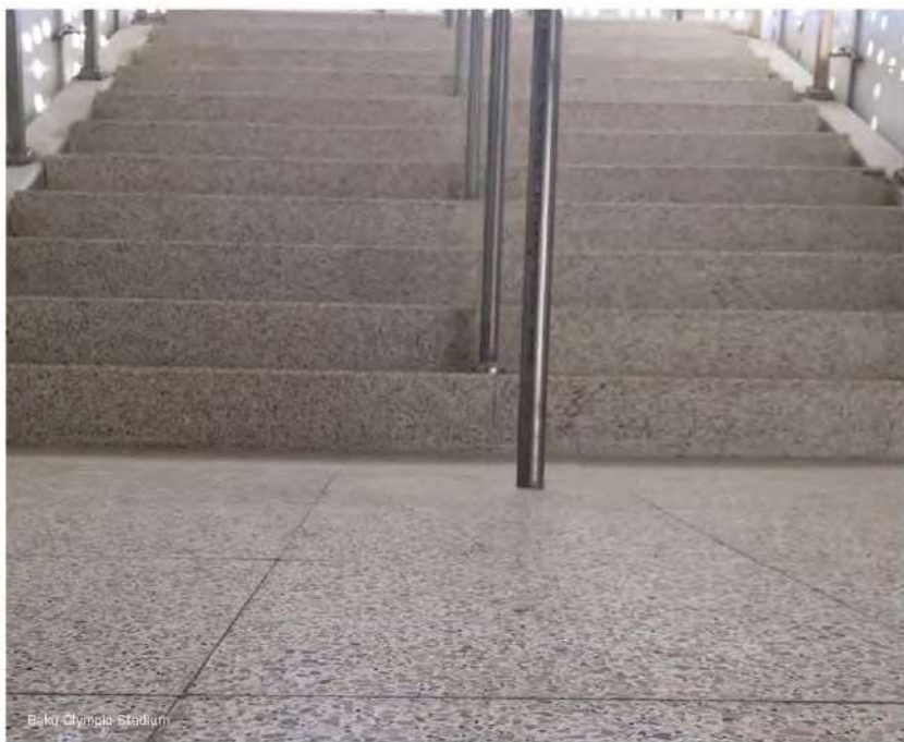
Baku Olympic Stadium
