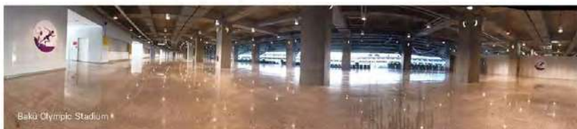
Baku Olympic Stadium
